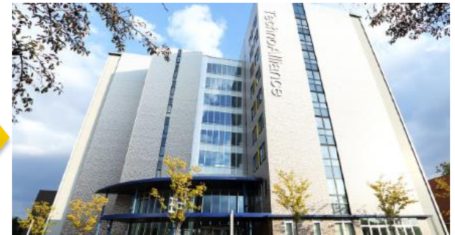
Techno-Alliance Building Research Alliance Laboratory (Daikin)
